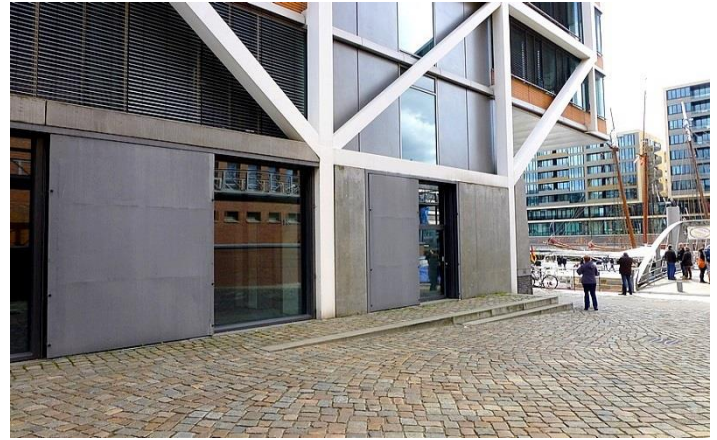
Hamburg: steel bulkheads can be closed to protect the windows of apartment blocks along the Sandtorkai
