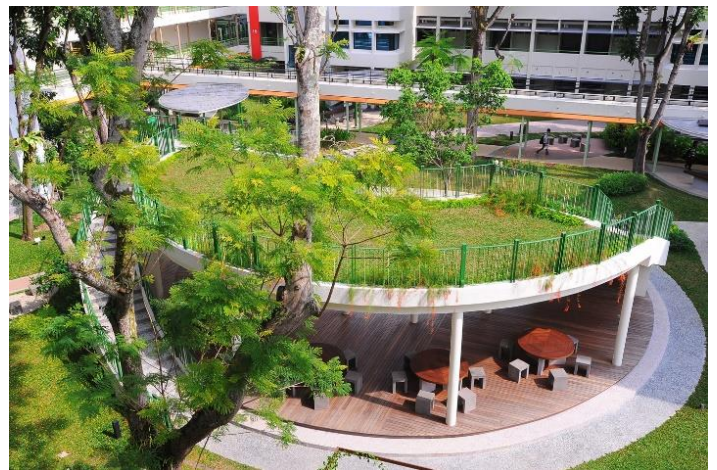
Elmich Green Roof and Rain Water Harvesting at Singapore Polytechnic
