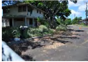
Abandoned Navy housing area adjacent to station – potential TOD opportunity site
