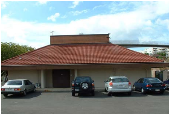
City's Traffic Management Center.
