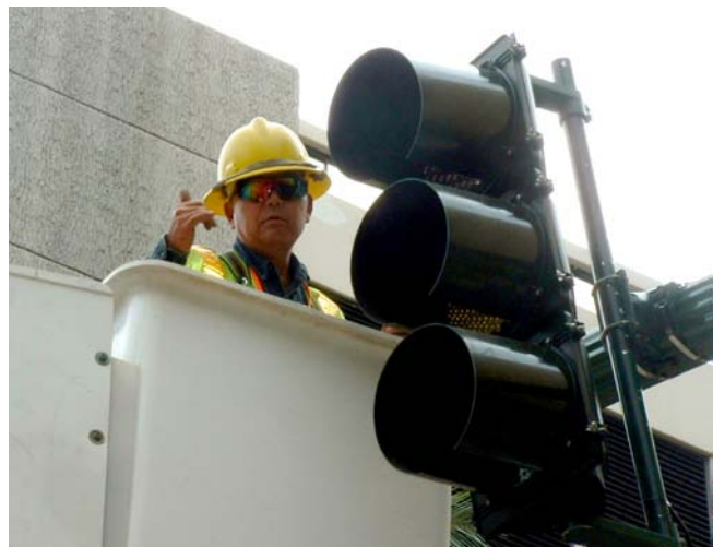
Traffic Signal Electrician repairing a signal light.
