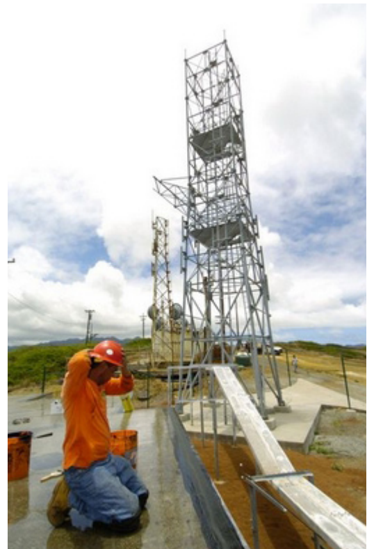
Construction at the Koko Head facility.
